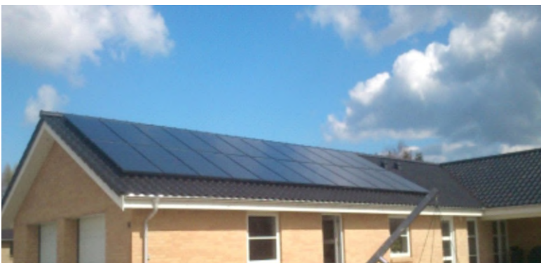
Denmark 6KW Home On-grid System
